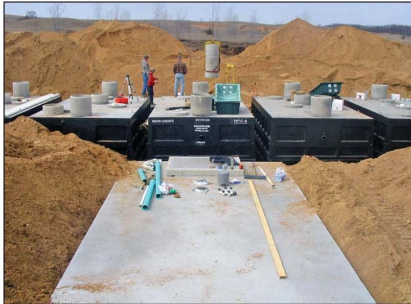
At left, the lid of the equalization tank in the foreground and the five 9,000-gallon treatment tanks, each with a 9.0 FAST unit, in the background. Below, Bill Bergh with the Orenco control panel.
