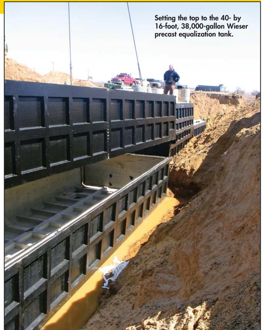
Setting the top to the 40- by 16-foot, 38,000-gallon Wieser precast equalization tank.
