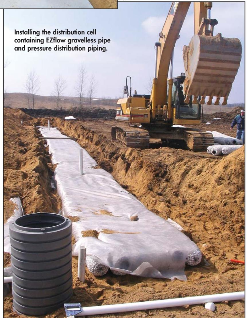
“The biggest reason for the four zones was that it allowed us to keep our pump sizes down,” says Bergh. Every time a pump shuts off, effluent drains back from the absorption bed and flushes the effluent filter.
