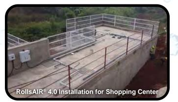
Settling Zone: After the MyTEE<sup>®</sup> Vault, the waste water flows into the RollsAIR<sup>®</sup> "Extended Aeration" treatment zone.
