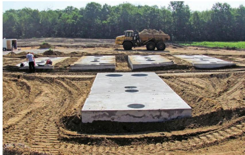
The flow equalization tank with the four FAST treatment tanks behind it. (Photos courtesy of Clear Water Environmental Systems)
